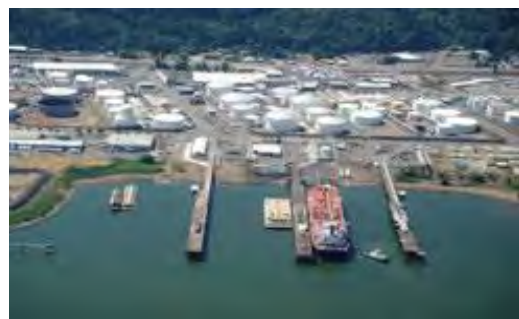
Critical Energy Infrastructure Hub, Willamette River
